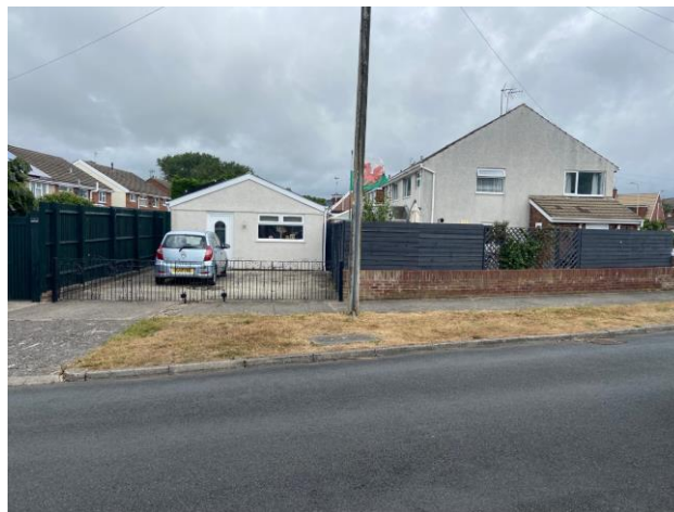
Fig. 6 - The existing driveway to be widened
